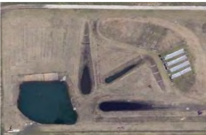
Figure 1. The field research and demonstration site shown in this aerial view includes an earthen berm, a detention pond, and three channels of varying configurations.
