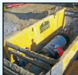
STEEL TRENCH BOX
