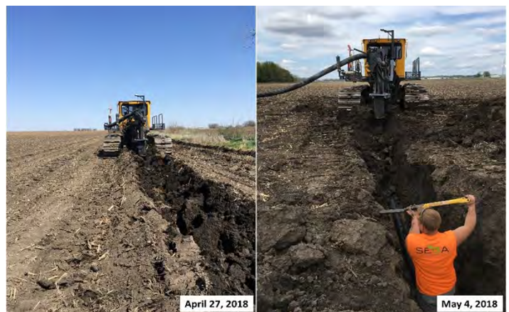
Figure 1. Tile installation in the monitoring fields
