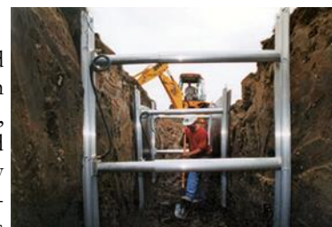
Credit: Pro-Tec Pro-Tec installing shoring
