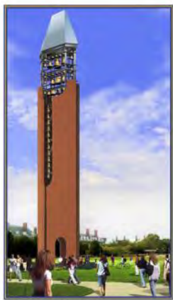
View of Bell Tower looking to the Northwest
