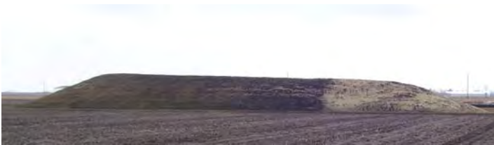
(upper right) One of the sediment collection ditches at the erosion control testing site; an example of the kind of problems this site will help correct; (left) The berm in early March, 2010.
