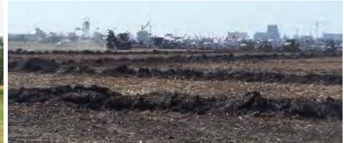
RCCF Tile Installation Demo
