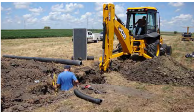
(r to l) Cold refreshments for a very hot day; Crowded dining room at Edgewood; Ryan Maltby and Sievers Equipment Co backhoe prepare to install the control structure; Hydramaxx wheel trencher gets ready to lay one of the saturated buffer tile lines; Control box in place and plumbed for the next rain.
