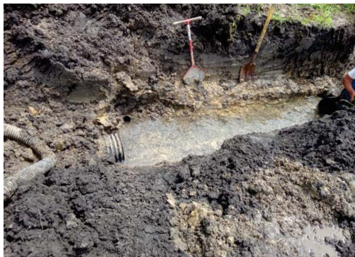
Figure 4. Repairing old clay tile impacted by new drainage system
