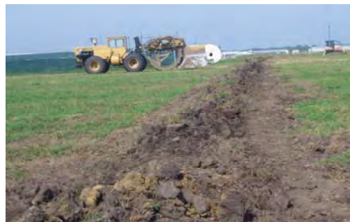
Farm Progress Show tile installation project
